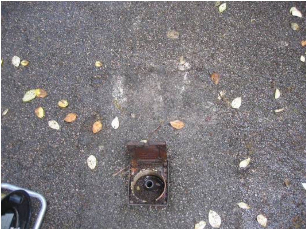
Plate 32 Scarborough South Cliff H5
