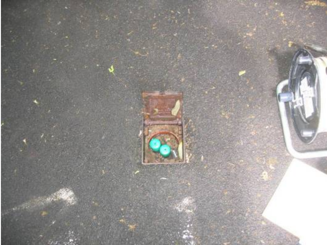
Plate 45 Scarborough South Cliff D2
